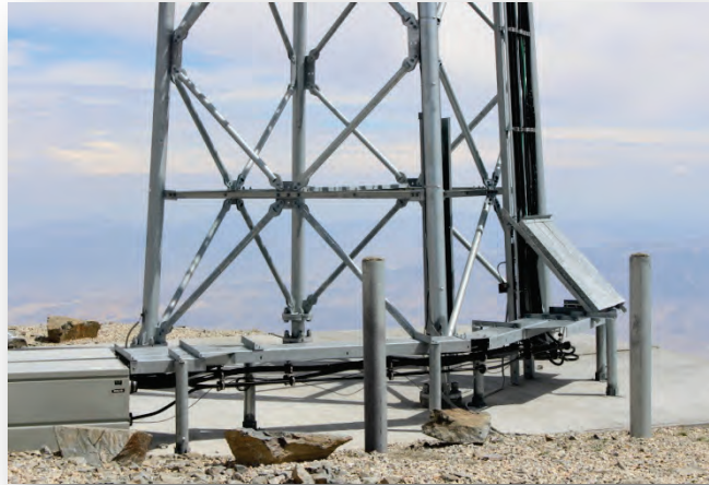
Figure 3-5. Above-Ground Raceway
